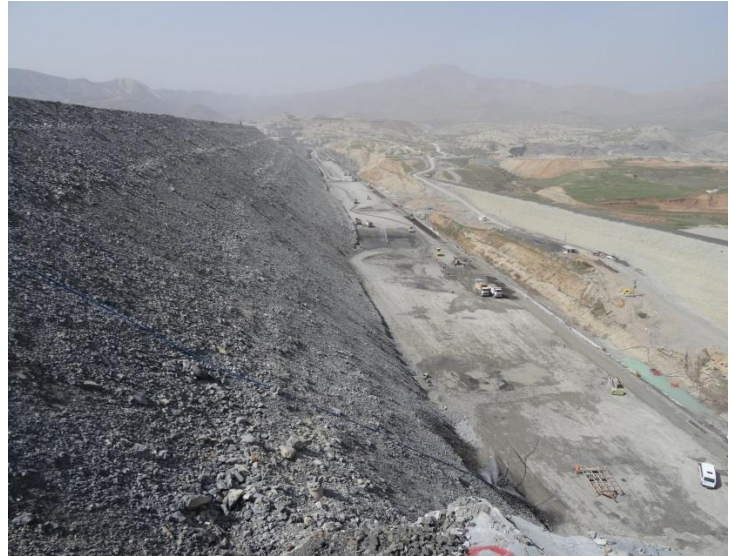
Upstream Dam filling works of CFRD Dam (March 2014)
