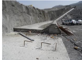
Curb and plinth construction of CFRD Dam
