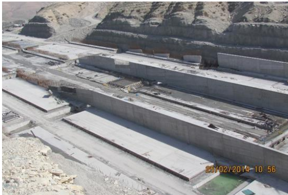
Spillway chute channel construction
