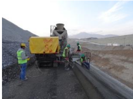
Curb and plinth construction of CFRD Dam
