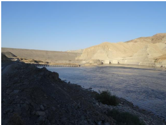
Downstream view of CFRD Dam & River Diversion tunnels
