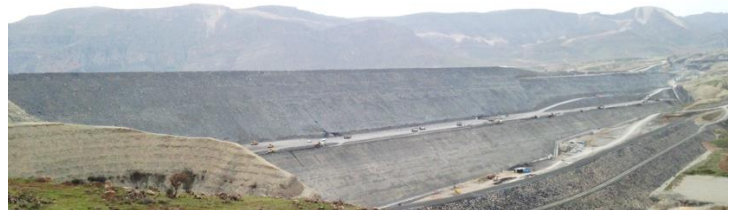
Upstream view of CFRD Dam / US Cofferdam (Dam filling 80% completed)
