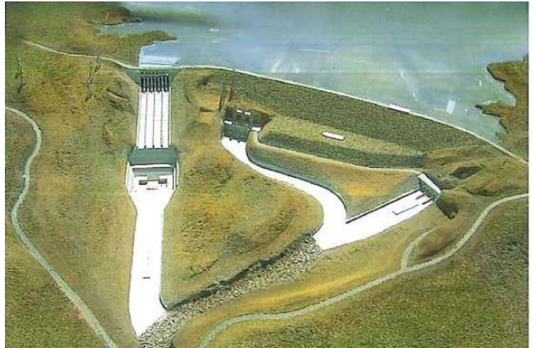
General overview of Ilisu Dam & HEPP with CFRD-Main Dam, Concrete gravity Dam, Spillway, Power Intake & Tunnels, Powerhouse, Diversion tunnels with Low Level Outlet
