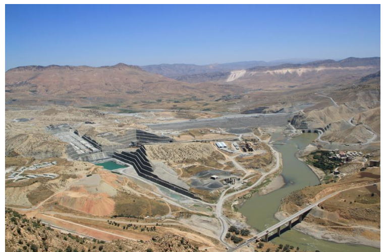
General overview of Ilisu Dam & HEPP from Downstream (Dec. 2013)
